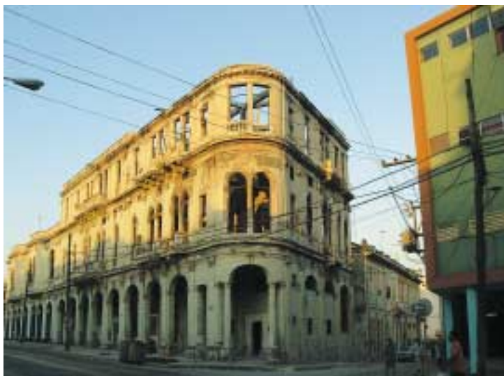
The colonial palaces of Havana fall apart. Several collapse every day.
