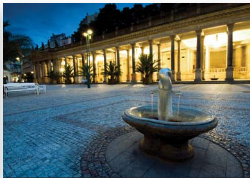
Mill Colonnade, Karlovy Vary
